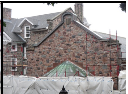
Sherriff Hall – windows, precast, pointing, flashing (24 visits Jun 6 to Sep 12, ongoing work)
